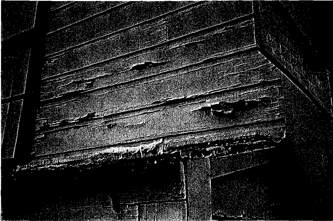
Paint Failure on Bungalow M-5
