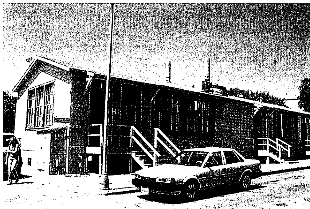
Bungalows, installed in 1957, formerly used as military barracks in World War II, located on the east side of the campus.
