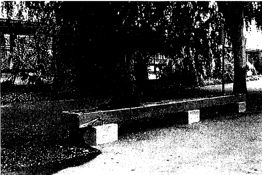
Seating northeast of the student park outside of classroom building shows signs of wear.
