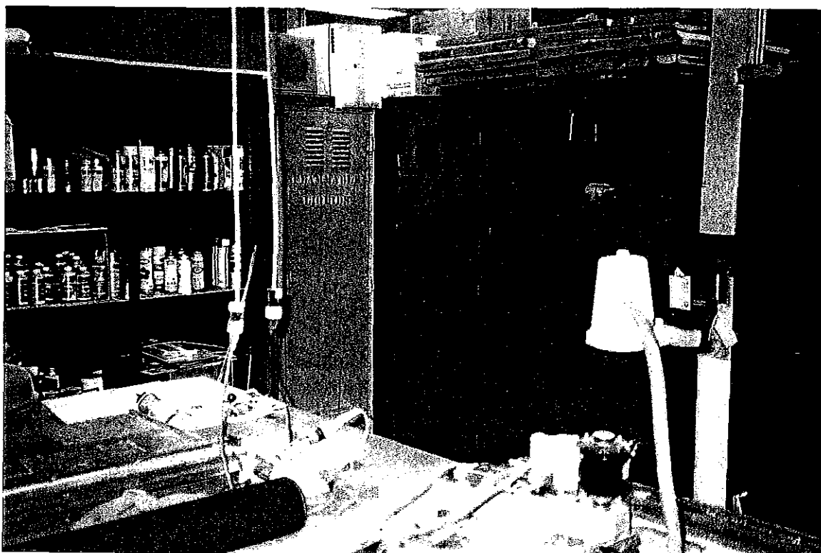
Flammable Materials Storage Cabinet
