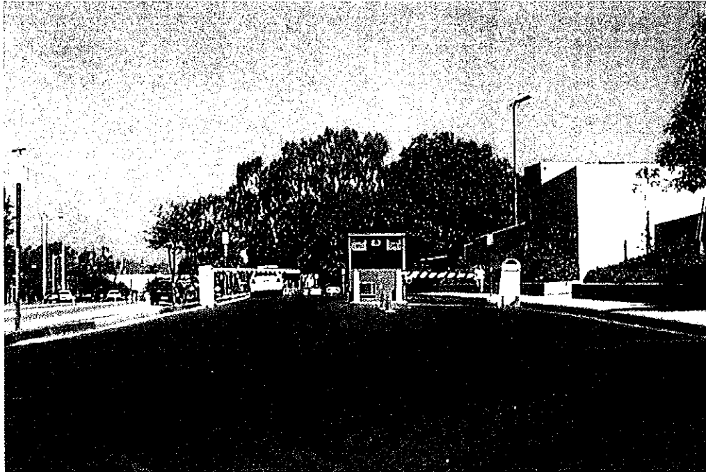
View looking east along Avenida Cesar Chavez. Guard Booth is on frontage access road on the north side of Avenida Cesar Chavez.
