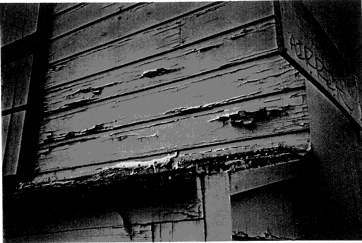
Paint Failure on Bungalow M-5
