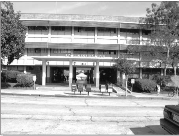
View of administration building looking east from Heliotrope Drive.
