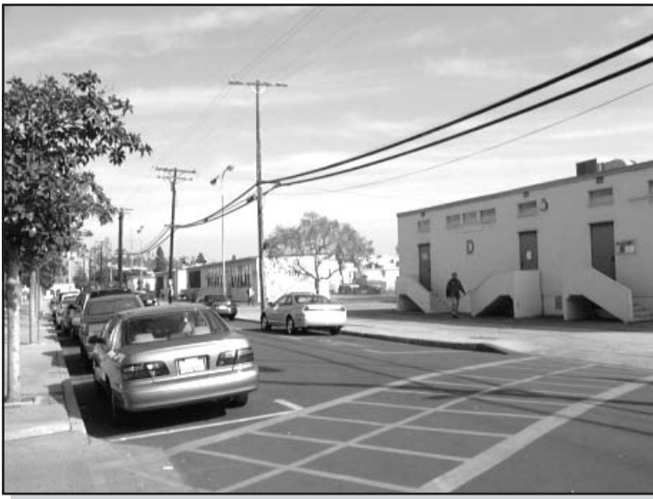
Bungalows along Monroe targeted for demolition.
