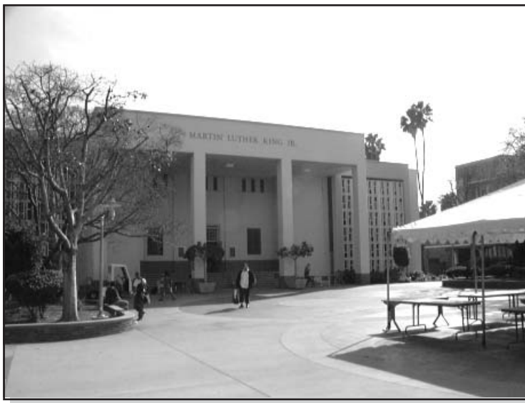
Martin Luther King Jr. Library targeted for demolition. New library will be located at the northern edge of the campus boundary at Willowbrook Avenue.
