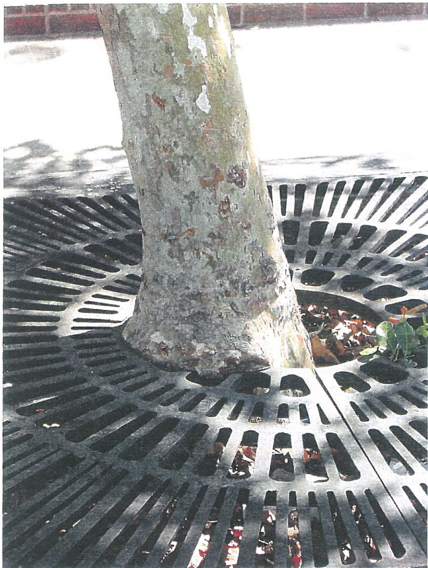
This tree grate has become imbedded in the base of this plane tree. Besides weakening the base, it will be further damaged by removal.
