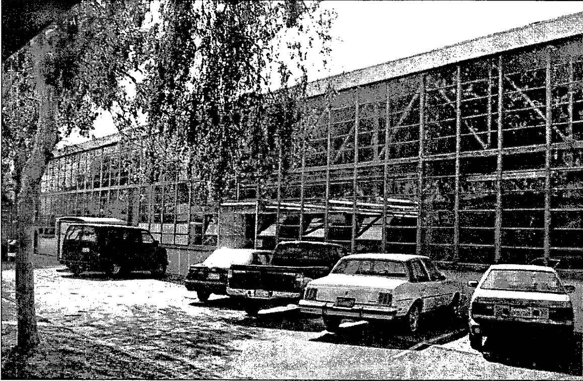
Figure 3-18: Tech Building 1, North Façade
