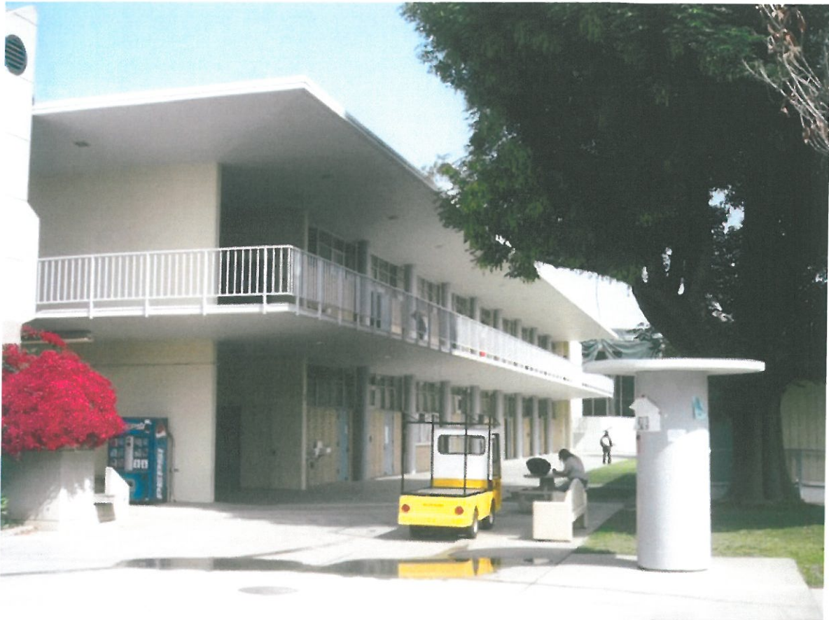
Figure 4 Science Building to be Demolished
