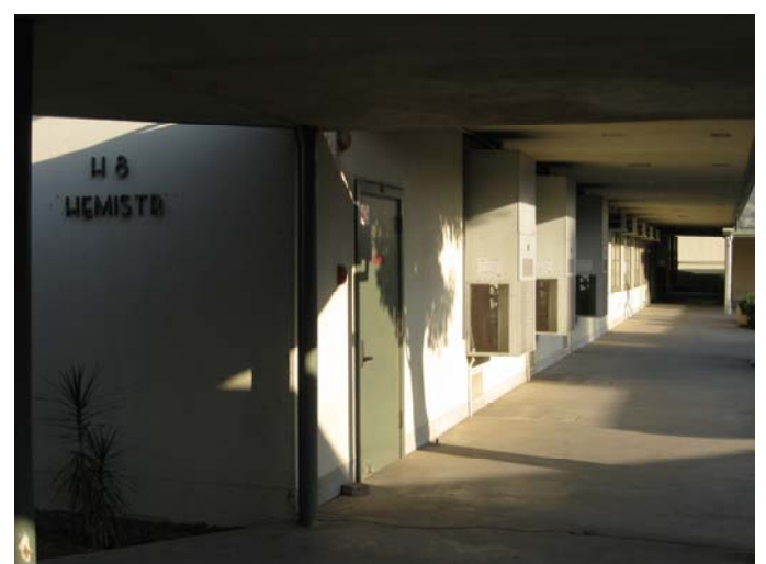
Building H8 Overview (Southeast)
