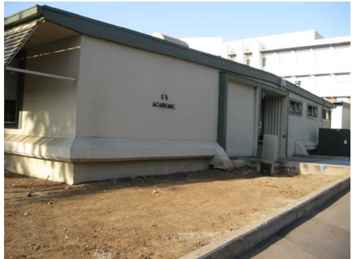
Building E5 Overview (North)
