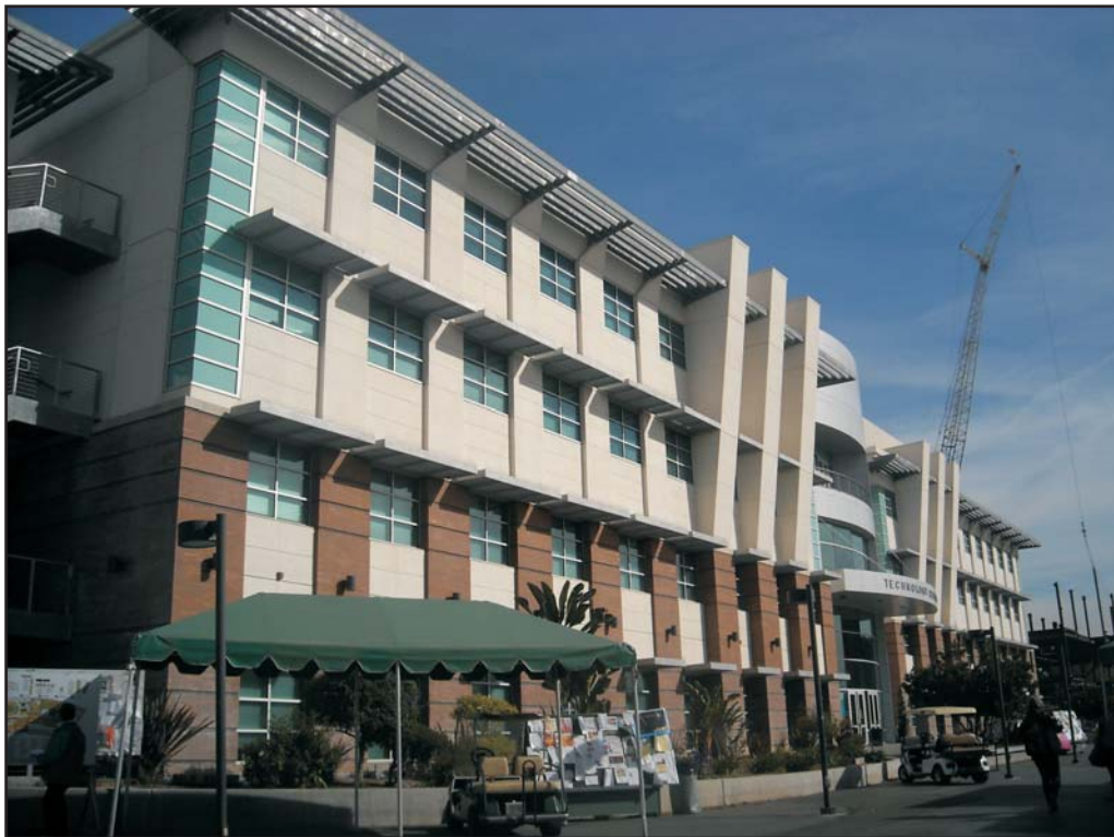
Technology Center. Light beige concrete, brick and glass exterior, flat and curved facade with a flat roof and symmetrically spaced window openings.
