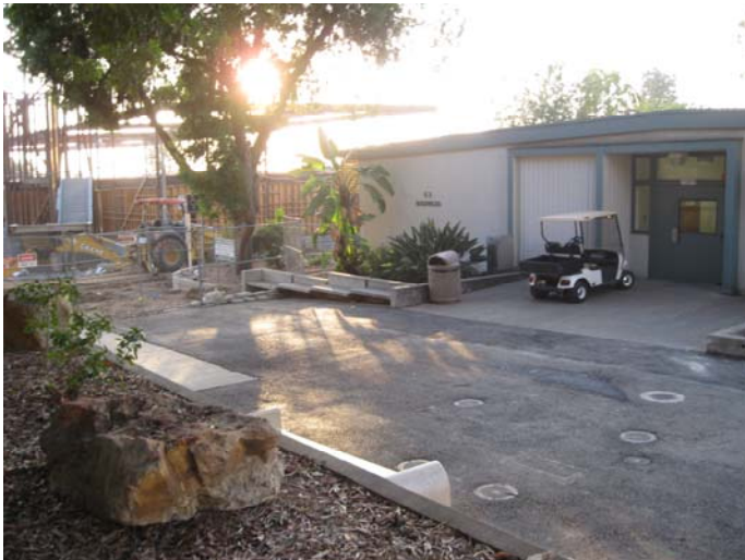
Building E3 Overview (Southwest)
