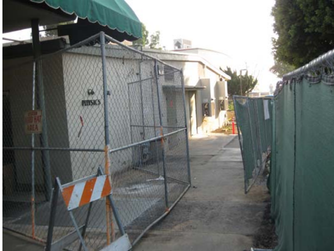
Building G6 Overview (Southeast)
