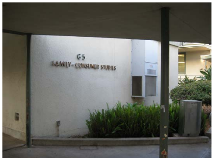
Building G5 Overview (Northwest)
