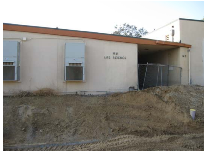
Building H6 Overview (West)
