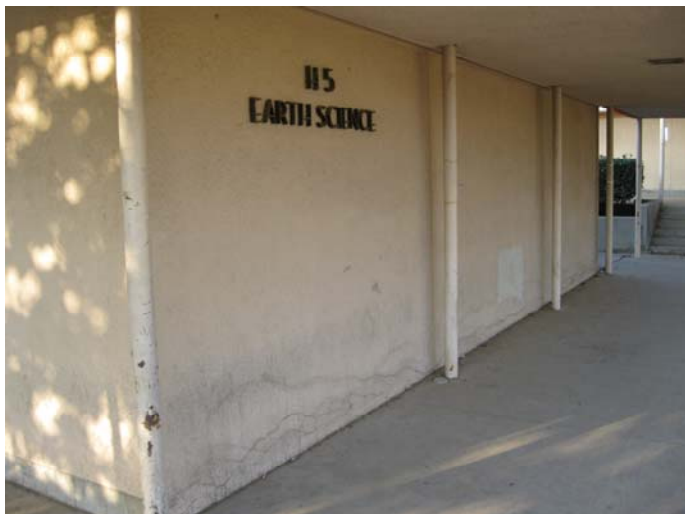
Building H5 Overview (Northeast)
