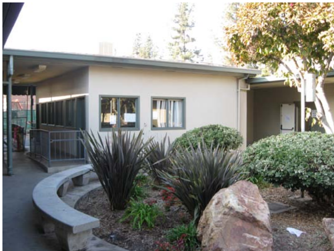
Building H7 Overview (East)
