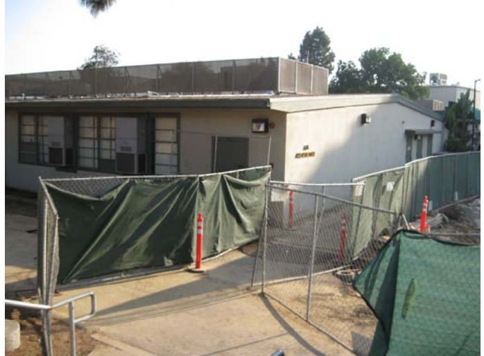
Building G8 Overview (Southeast)
