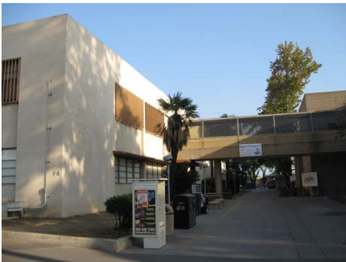
Building F5 Overview (Northeast)
