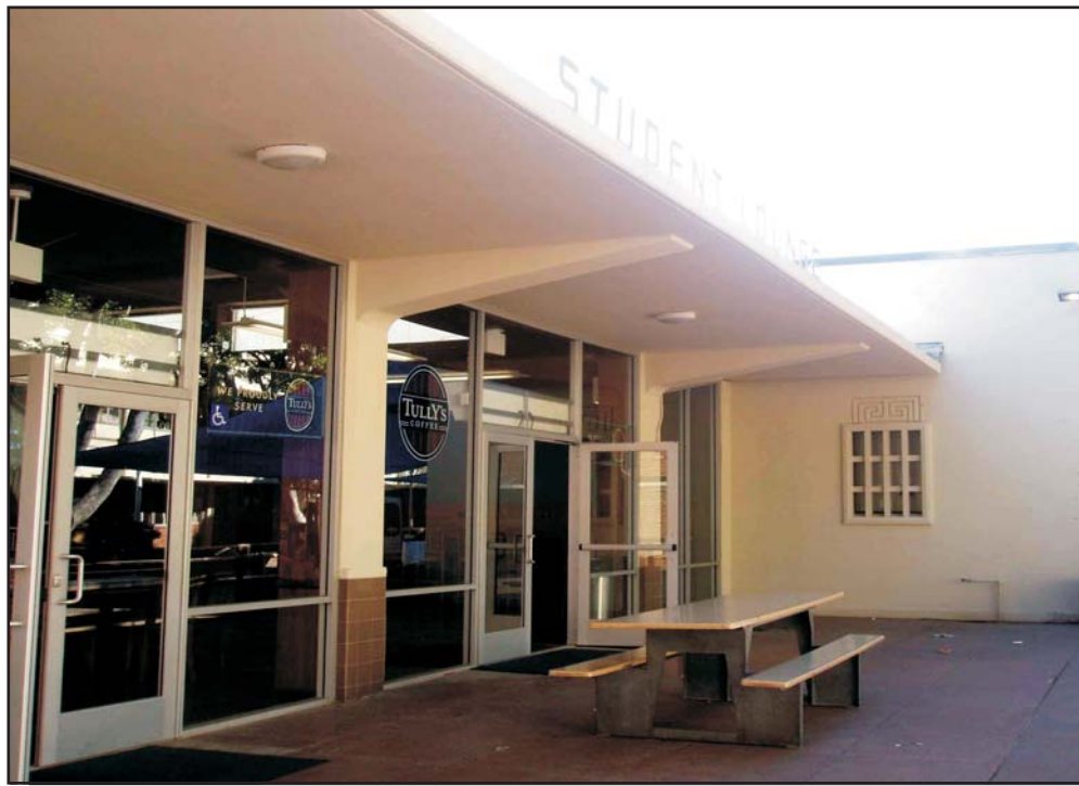
View of the addition to the northeast end of the Cafeteria.
