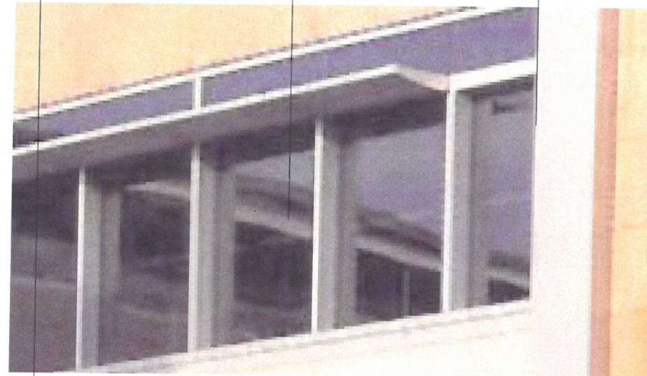
Solid sun shade integrated into window system
