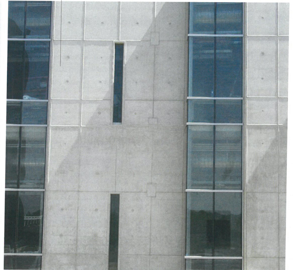
Exposed cast-in-place concrete with expressed detailing
