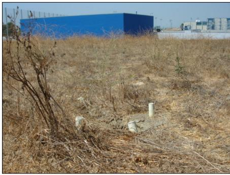
View of a possibly abandoned or damaged monitoring well in northwest portion of the target property
