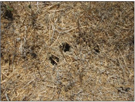
View of rodent holes observed in soil above cap
