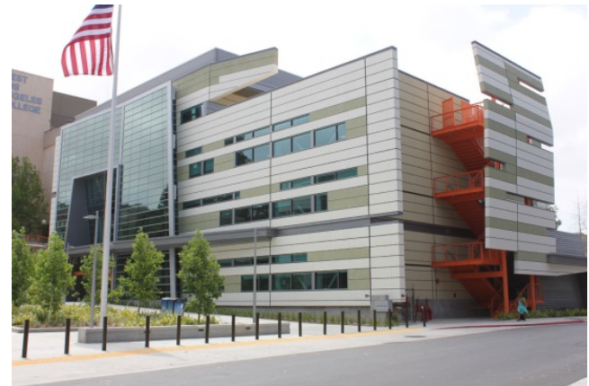
The General Classroom (GC) Building is a four-level building near the center of campus and accessible from 'B' Street. It contains classrooms and office space.
