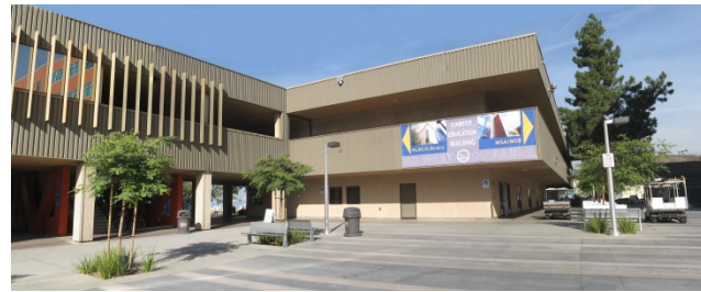
The CE Building is a two-level classroom and office building that connects to the HLRC via an enclosed, sun-screened bridge.
