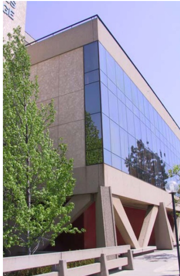
The HLRC Building is a four-level structure that houses the library and learning center. It was one of the first buildings on the West Los Angeles College campus.
