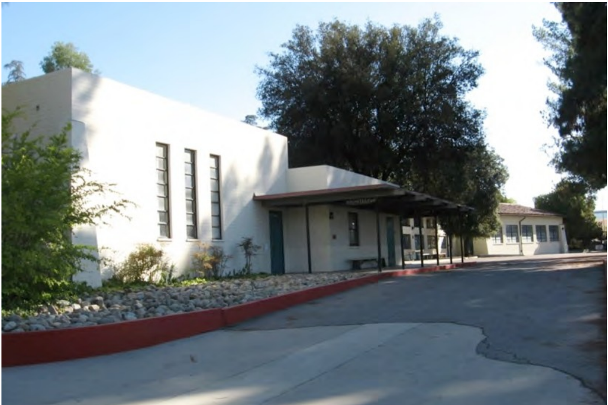
Photo 1: 3800 Building (Applied Technology), Full Overview, Looking Southwest
