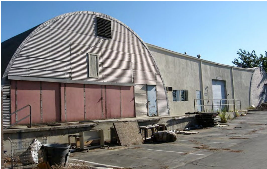
Photo 5: View, Exposition Hall Quonset Hut, Former Facility Maintenance Yard, Looking Southwest
