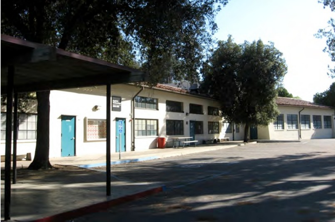
Photo 2: View, 3800 Building (Applied Technology), Looking Southwest
