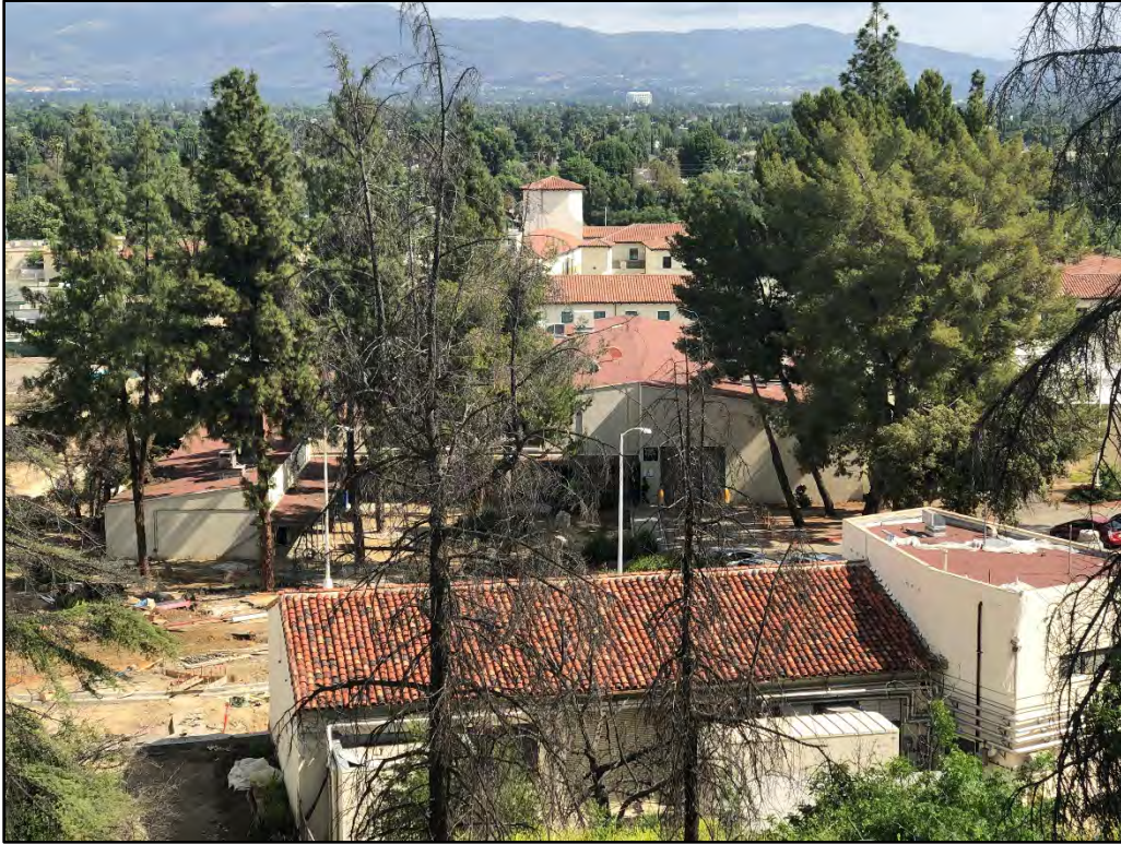
Photo 5. Applied Technology Building, foreground (to be demolished)
