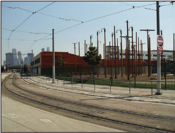
View 1: View looking northeast up Flower Street toward Parcel 2 (red building).
