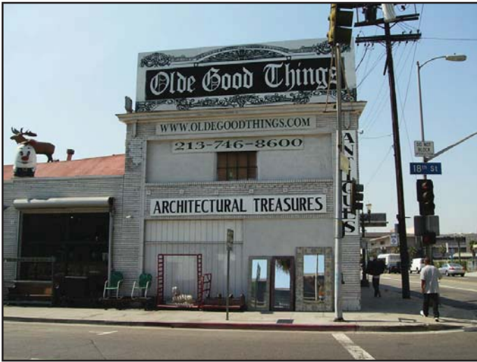
View 5: View looking southwest across W. 18th Street toward retail uses on Parcel 4.
