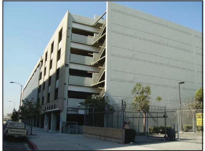
View 7: View looking southwest from Olive Street at one of the LATTTC's parking structures.
