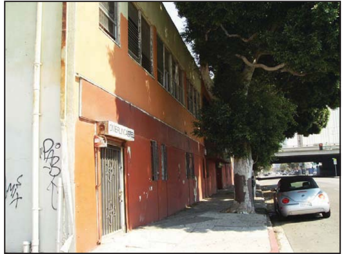
View 8: View looking northeast along Olive Street toward Parcel 4.
