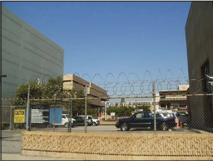
View 6: View looking northwest toward the existing LATTTC campus from Olive Street.
