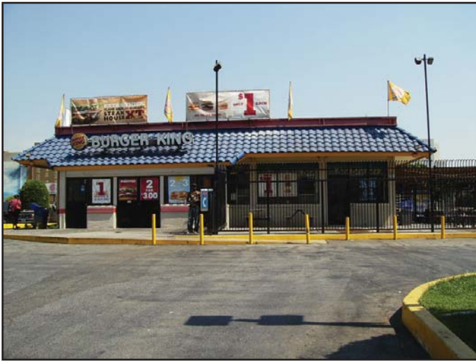
View 1: View looking northeast from Washington Boulevard toward Parcel 4.
