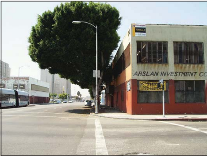
View 7: View looking southwest from the intersection of W. 18th Street and Olive Street toward Parcel 4.
