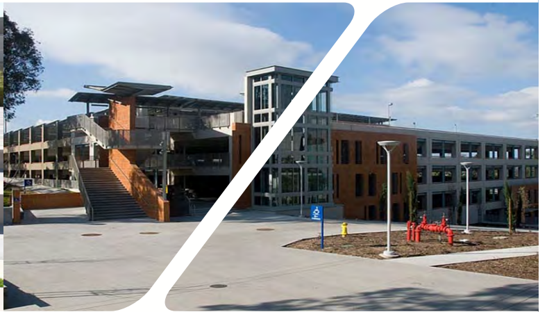
Parking Structure - Lot 8
