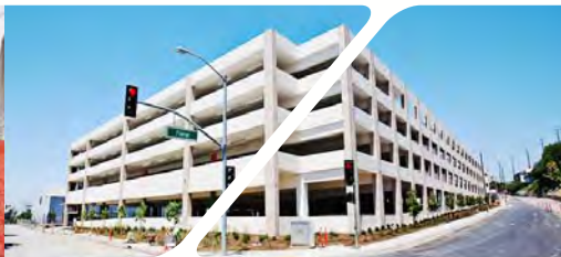
Parking Structure Lot 4
