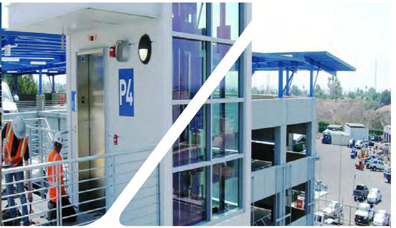
Northeast Quadrant Parking Structure
