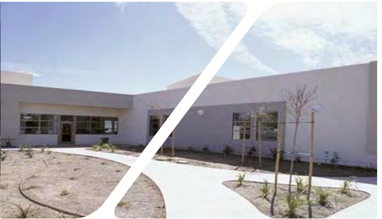
Maintenance and Operations, Sheriff Station
