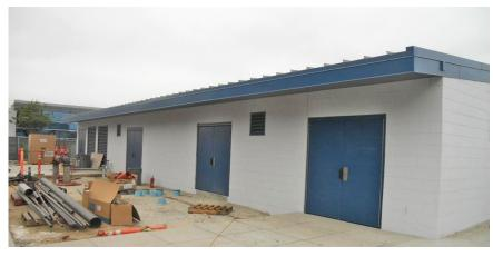
This is the Pump House and Fire Water Upgrade project. The project will construct a new pump station and add new fire and domestic water lines. This project is under construction.
