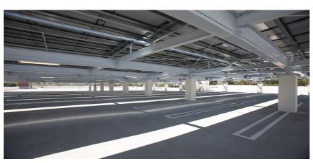
This project installed 97,000 square feet of photo-voltaic carport canopies throughout student/staff parking lots on campus. The project allows the college to produce 2,260 kW of power. This project is complete.
