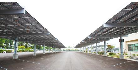
This is the Solar Energy Parking Lot and Internal Roads project. The project is comprised of the photovoltaic panels for Lots C, D, M&O and the Parking Lots/Internal Roads Parking Lot D. There is 1,022.14 kWdc (4,172 PV Panels) total for this project and is it is divided across the parking lots. The division is as follows: Lot C = 51.45 kWdc = 210 PV Panels, Lot D = 816.34 kWdc = 3,332 PV Panels and M&O Lot = 154.35 kWdc = 630 PV Panels. This project is under construction.
