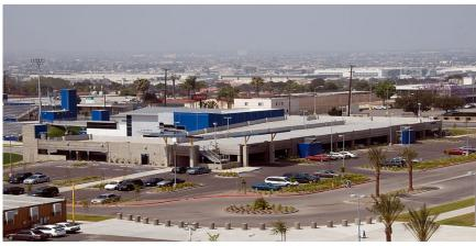
This is the West Entry Drive and Parking Lot Facilities project. The West Entry Drive has 507 parking spaces, including site improvements to the existing West Entry Drive and the Parking Lot facilities in the northwest corner of the campus. The parking structure is a 128,982 square foot multi-level (3 levels + roof) structure. The parking structure consists of 412 parking spaces with another 95 spaces on grade, just north of the structure. This project is complete.
