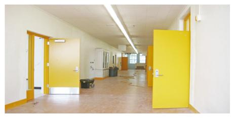
This is the Life Science Renovation Project. This project renovated the Life Science building for instructional and office space. Improvements will include: ADA compliance upgrades, elevator upgrades, painting, interior wall reconstruction, and power/data upgrades. This project is complete.
