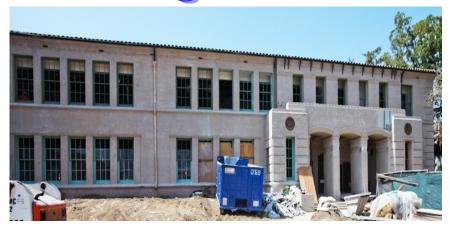
This is the Renovate and Modernize Building A project. The modernization will include interior/exterior paint, ceilings, restrooms, floors and infrastructure. The exterior will be restored to its original look. This is the only pre-1930's building that will be renovated and modernized. This project is under construction.
