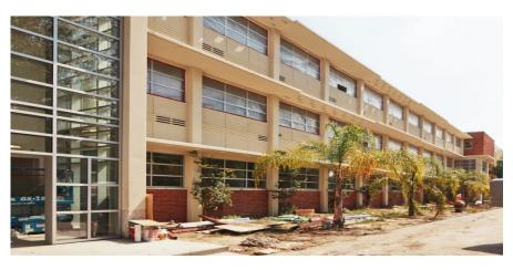
This project is the reconstruction of Jefferson Hall. The reconstruction provides a new configuration of classrooms, computer laboratories, and support spaces. The accessibility under ADA will be improved and hazardous materials will be abated. The utility systems (HVAC/electrical) will be upgraded to support technology use and enhance energy efficiency. Safety will be improved with a fire alarm upgrade that meets requirements for Division of the State Architect (DSA). This project is complete.
