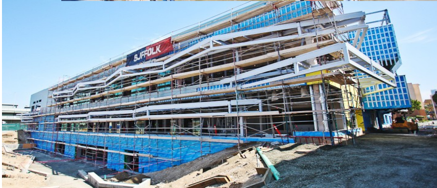
THE LEARNING ASSISTANCE CENTER RENOVATION PROJECT REPLACES THE BUILDING ENVELOPE, RENOVATES THE INTERIORS AND RECONSTRUCTS THE BASEMENT. THIS BUILDING IS SCHEDULED TO OPEN SPRING 2013.
