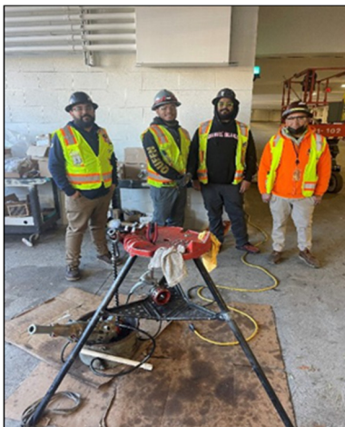
Nilsson Ramirez (second to right) Apprenticeship: LA Trade Tech CMU Program Local: IBEW Local 11 Contractor: Reyes Electrical Project: City College – IT Security and Sustainability Infrastructure
