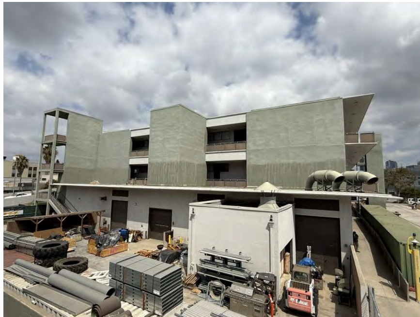
Photograph 4. Overview of south elevation, view north.
