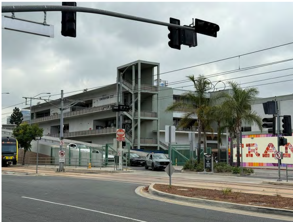
Exhibit 14. CMU Building (E2), west and south elevations, view northeast.
