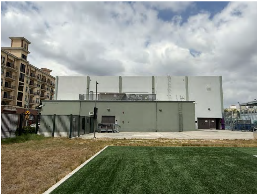
Photograph 4. Overview of east elevation (rear building), view west.
