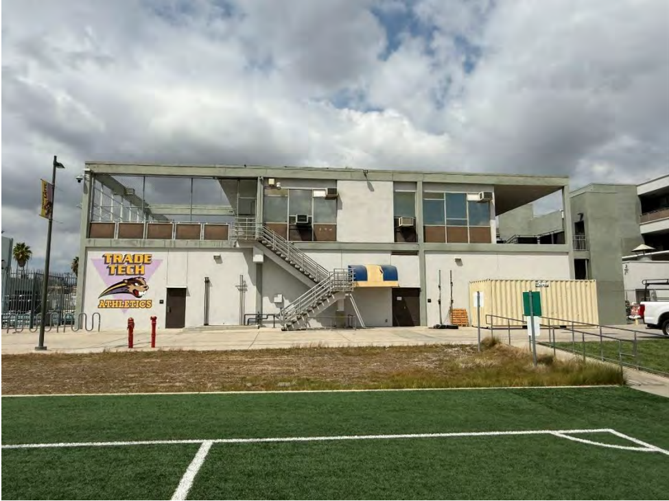
Exhibit 15. Athletics Building (F2) east elevation, view west
