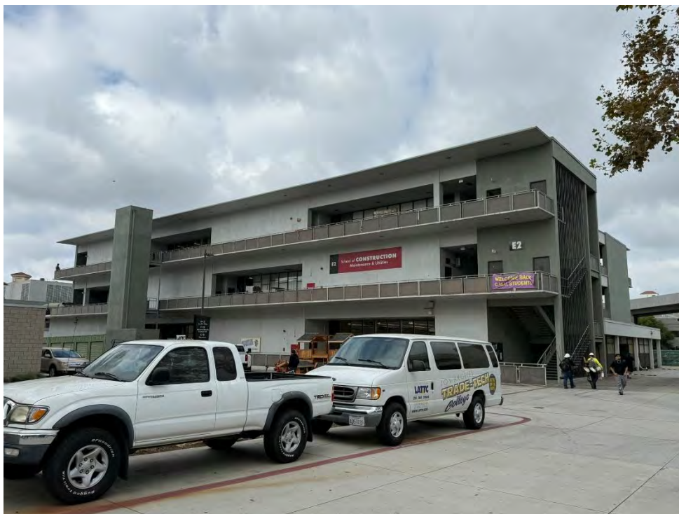
Exhibit 13. CMU Building (E2), east elevation, view southwest
