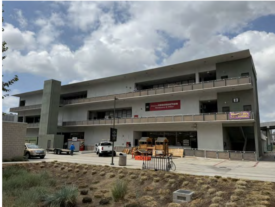
Photograph 5 1. Overview of east elevation, view west.
