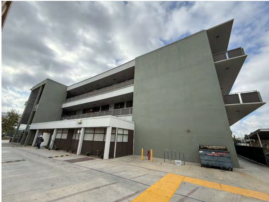
Photograph 2. Overview of north elevation, view southeast.
