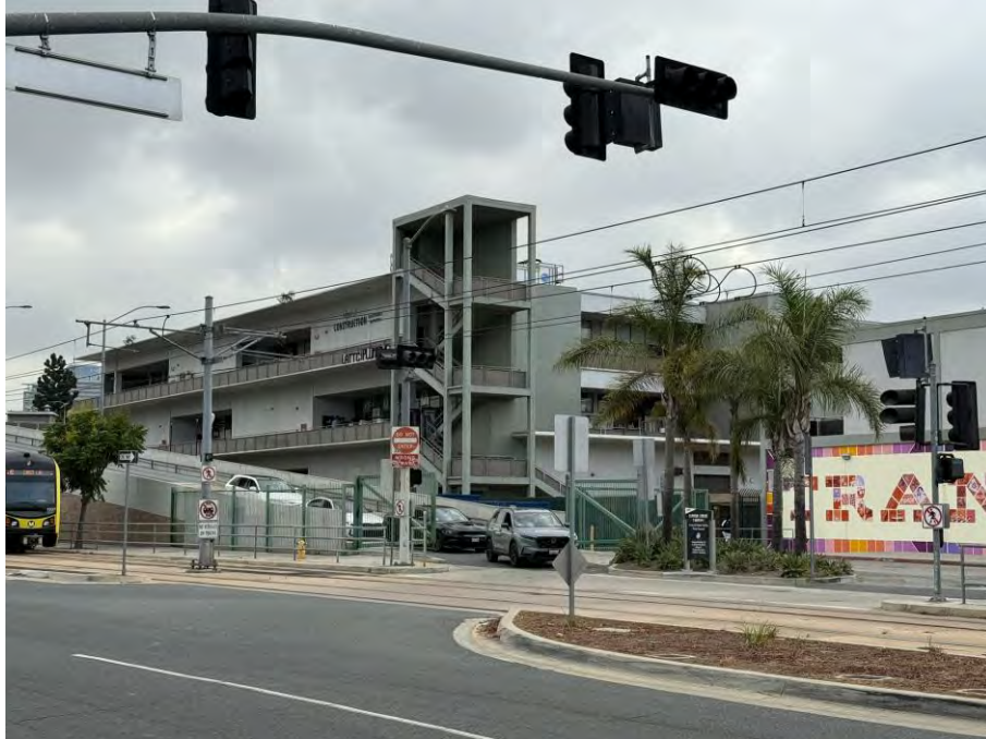
Photograph 3. Overview of west and south elevations, view northeast.
