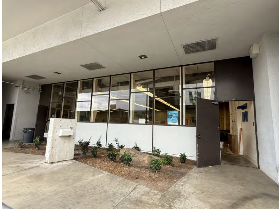
Photograph 7. Overview of windows and doors.
