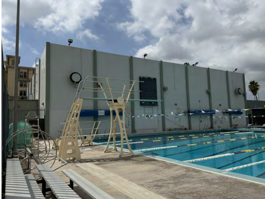
Photograph 3. Overview of north elevation, view southwest.
