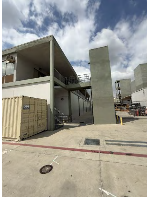
Photograph 5. Overview of elevator tower, view west.
