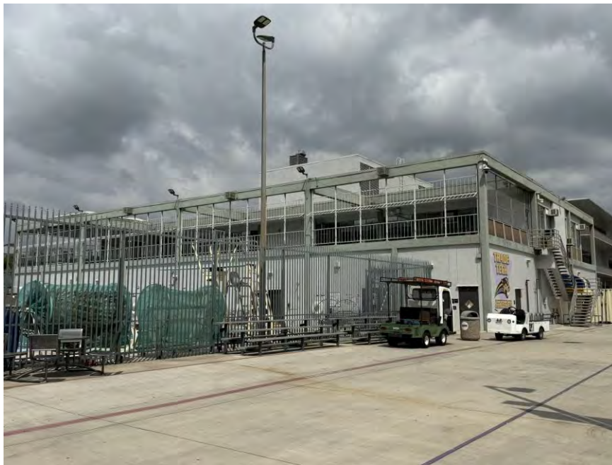
Photograph 3. Overview of south elevation, view northwest.
