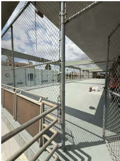
Photograph 4. Overview of south elevation corridor and atrium, view southwest.
