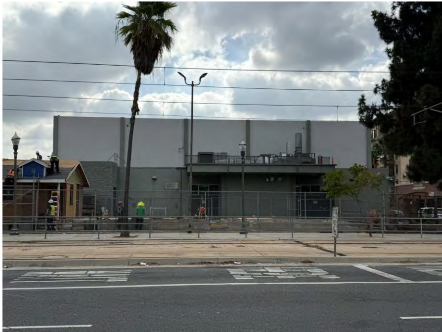
Photograph 2. Overview of west elevation, view east.
