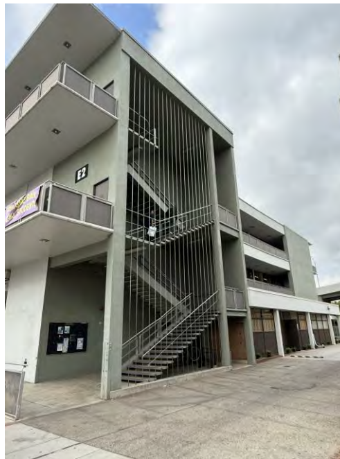
Photograph 6. Overview of northeast corner exterior staircase, view southwest.
