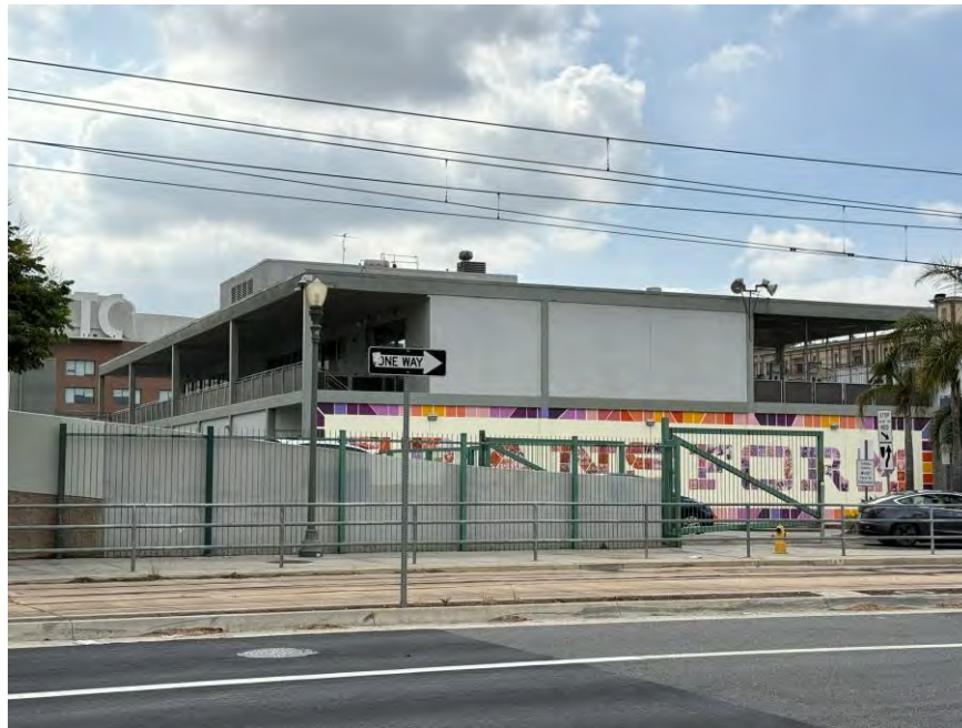
Photograph 2. Overview of west (rear) elevation, view southeast.
