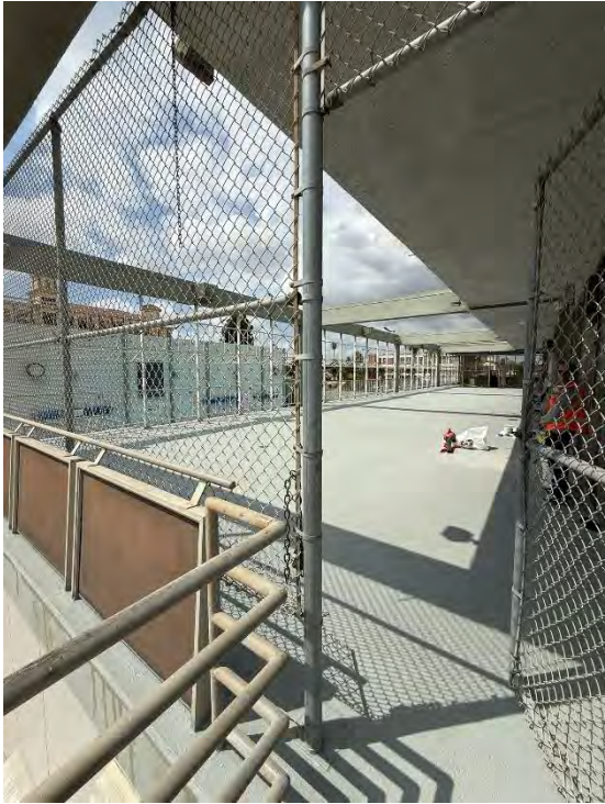
Exhibit 16. Athletics Building (F2), south elevation atrium, view southwest
